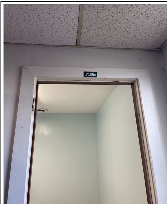
527-4 - AG Building - Room F100c
