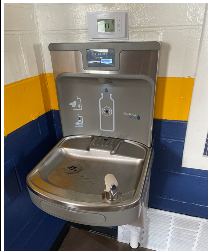
527-3 - AG Building - North Wall of Classroom
