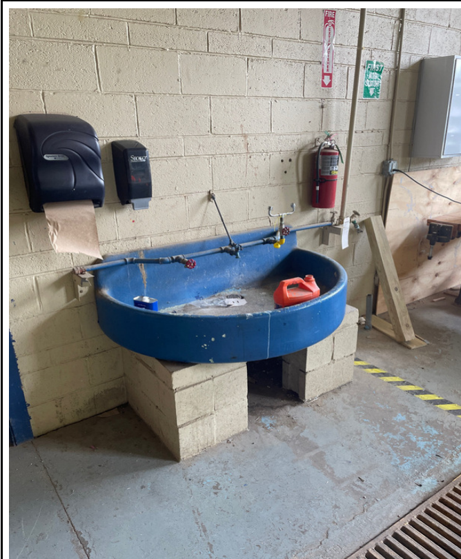
527-1 - AG Building - Shop East Wall
