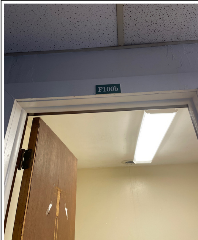
527-5 - AG Building - Room F100b
