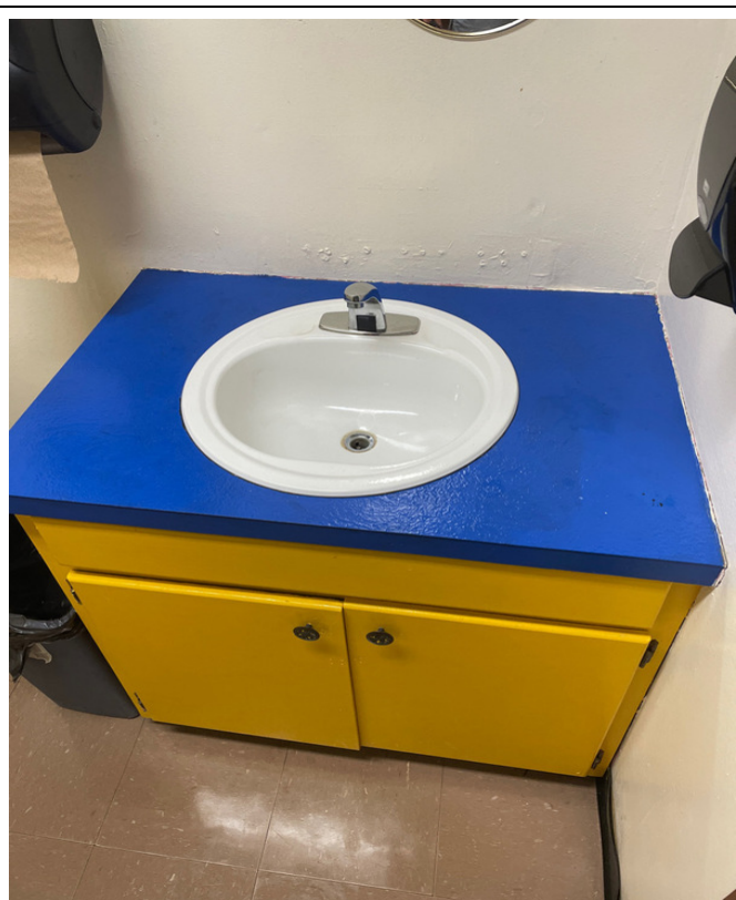
527-5 - AG Building - Room F100b
