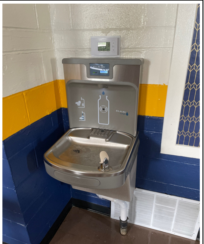
527-2 - AG Building - North Wall of Classroom
