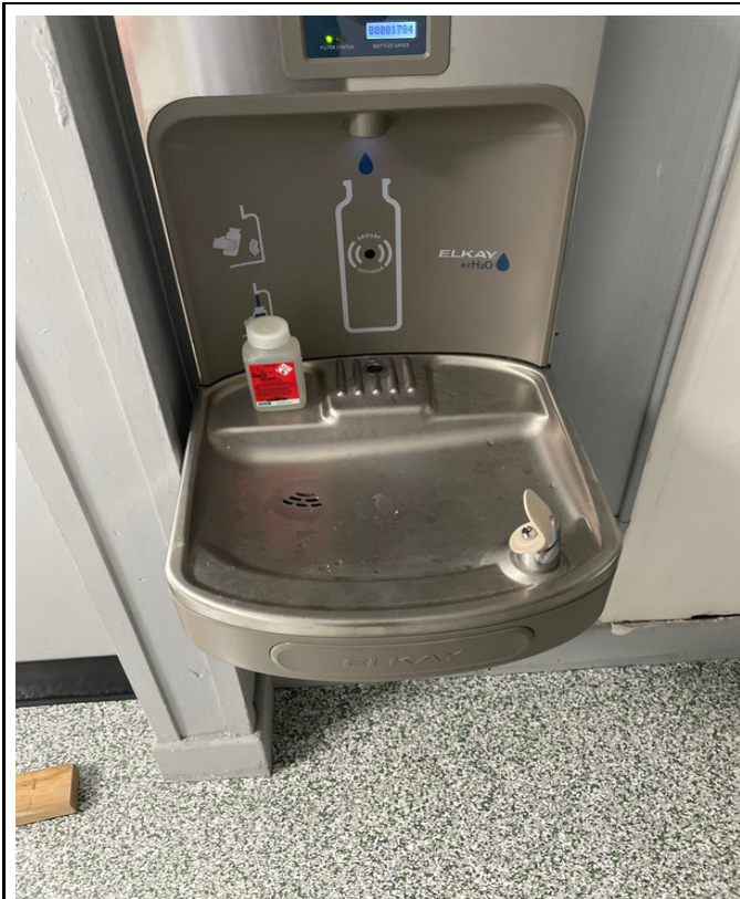
527-1 - 5th/6th Grade - Main Hallway
