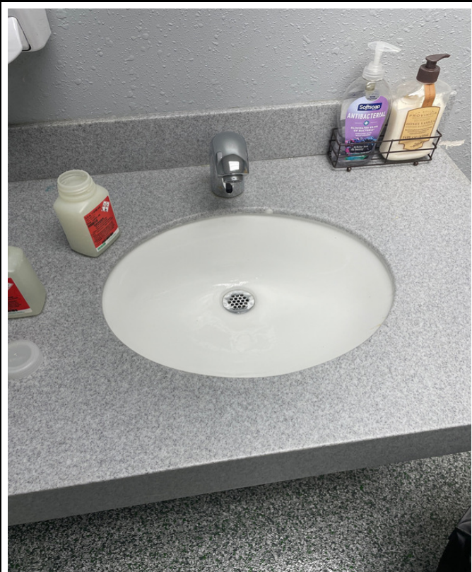
527-4 - 5th/6th Grade - Women's Restroom Right
