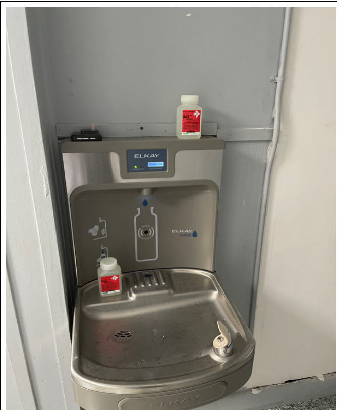
527-2 - 5th/6th Grade - Main Hallway
