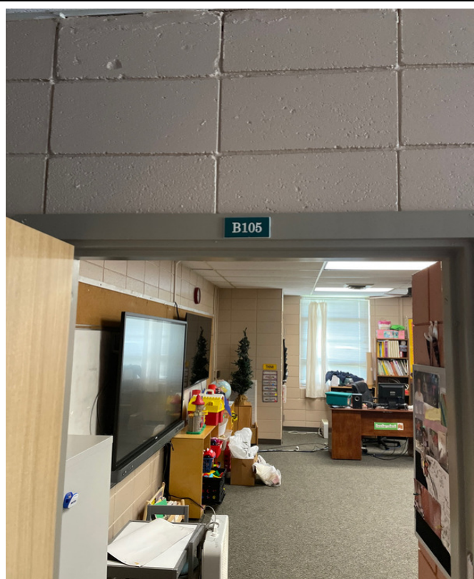
527-2 - Elementary School - Room B105
