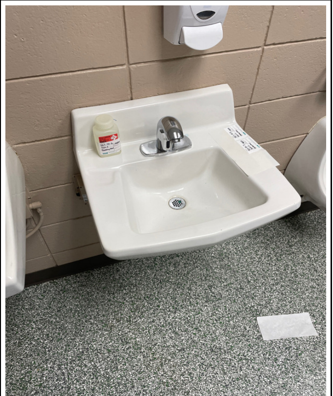
527-6 - Elementary School - Men's Restroom Right
