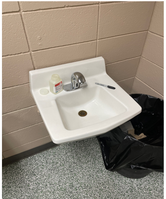
527-8 - Elementary School - Women's Restroom Right
