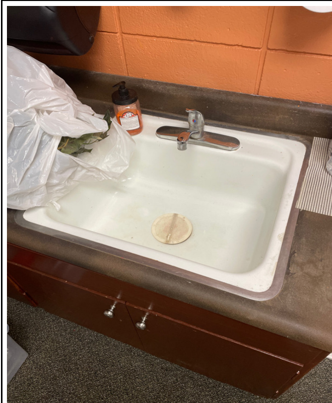
527-2 - Elementary School - Room B105
