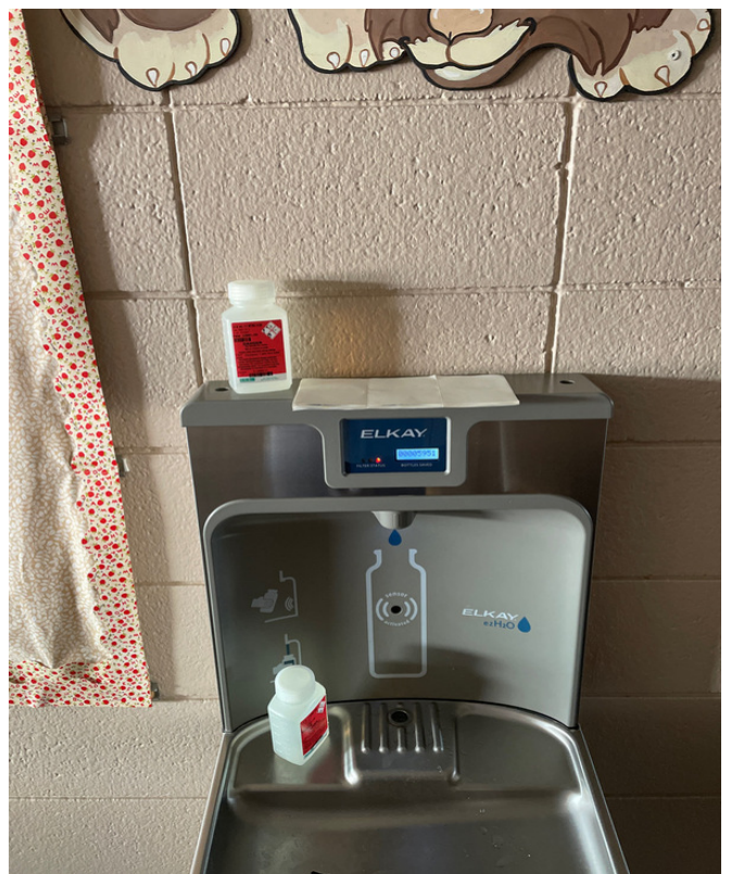
527-10 - Elementary School - Main Hallway South End
