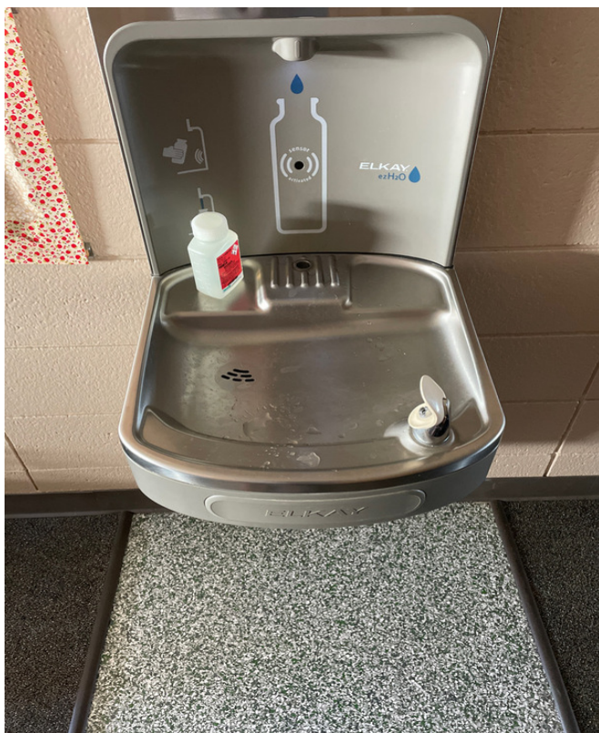
527-9 - Elementary School - Main Hallway South End
